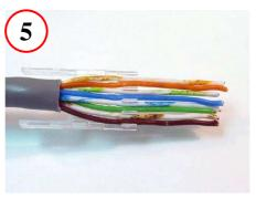
Insert each pair, being careful not to collapse ribs between each pair
