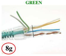
Untwist lower three pairs back to ends of side walls
